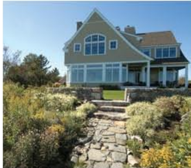
Builder Bob Reed's renovations completely changed the ocean-facing side of the house to allow 180-degree views.
